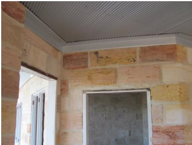
Ceiling above the front door. Photo G.Craig.
